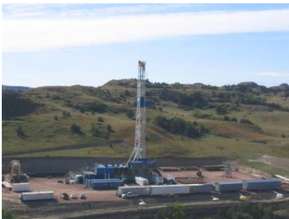
Nabors Rig 59 located in the Badlands southeast of Sather Dam
